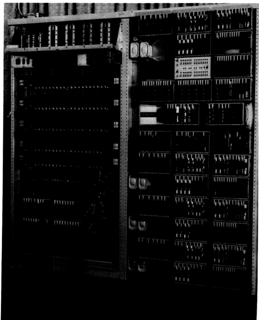
Fig. 3—Loop Testing Frame equipped with four MLT measurement modules.
